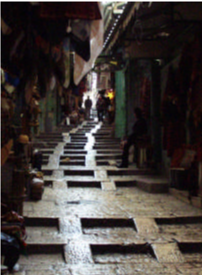
Old City stairs : These ramps match the spacing of vendor pushcart wheels – based on a standard that is centuries old! Preserved like the spacing of roman chariots: in US railroads.
